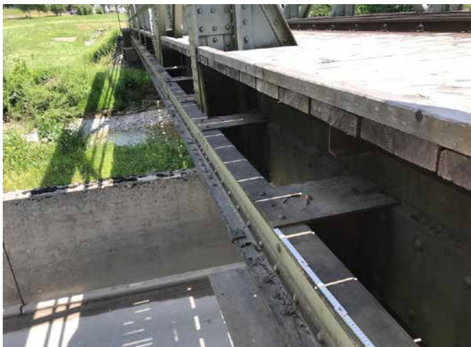
After the installation
