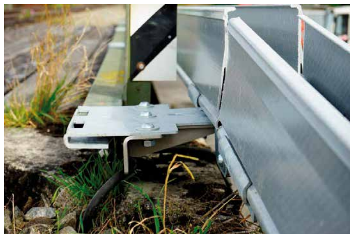
After the installation
