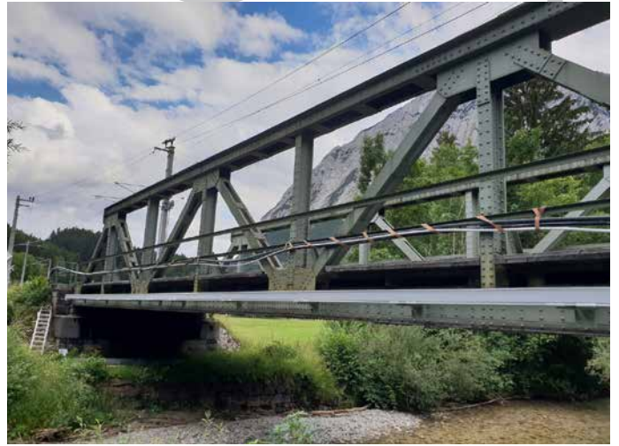
After the installation
