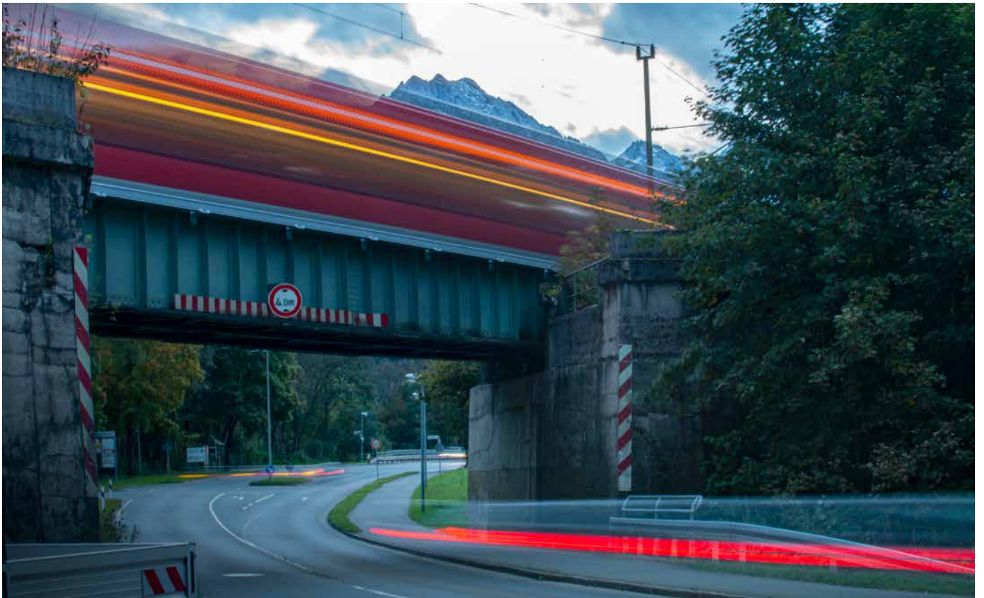
After the installation
